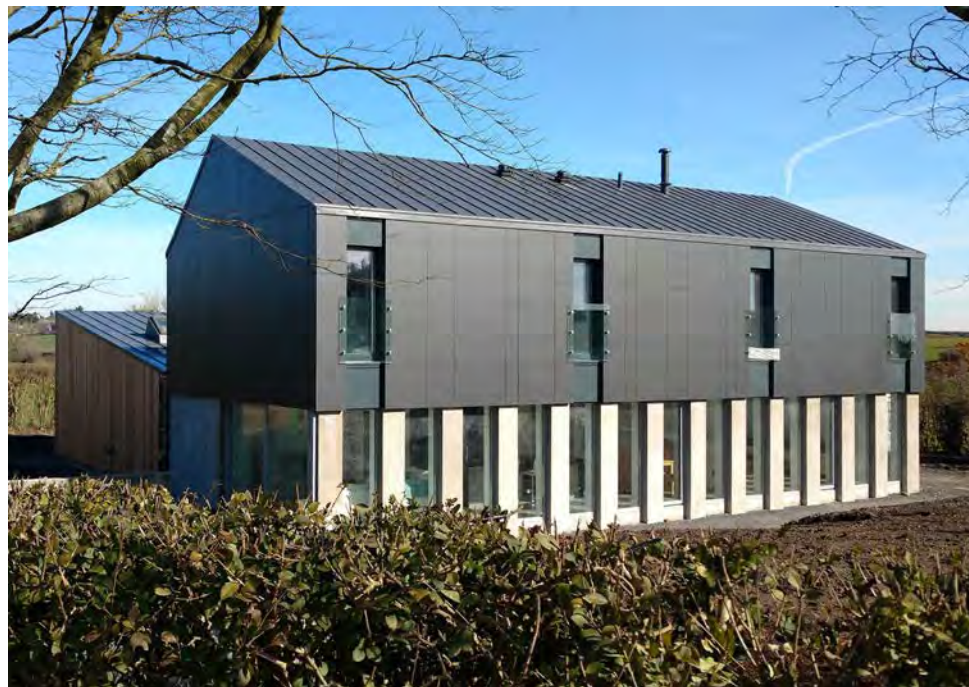
Example project with a fibre cement clad box on a glazed box, shaded by columns.
