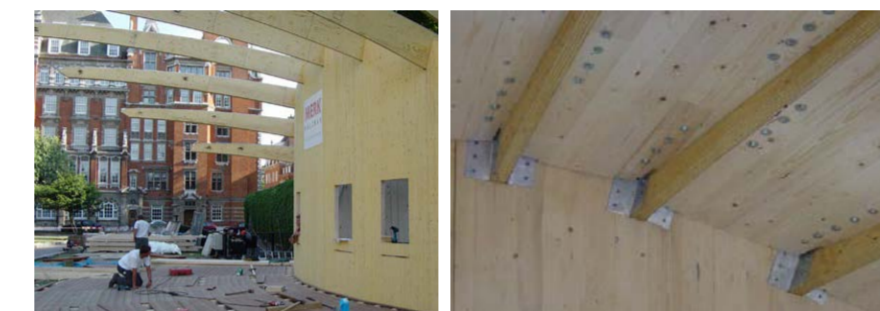
Picture 5: Cantilevered Kerto LVL Spruce roof beams, Picture 6: Roof Panels (Photos: PRS Architects)
