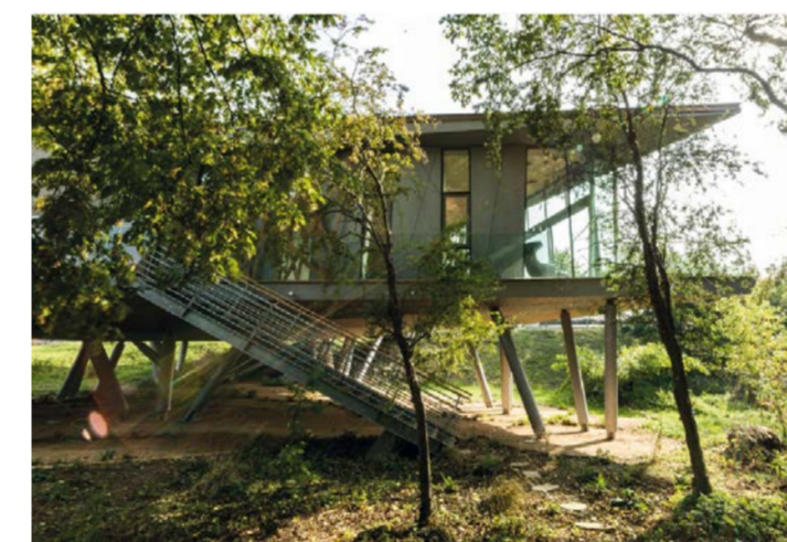
Picture 1: Rear view of building (All photos Julian Abrams)
