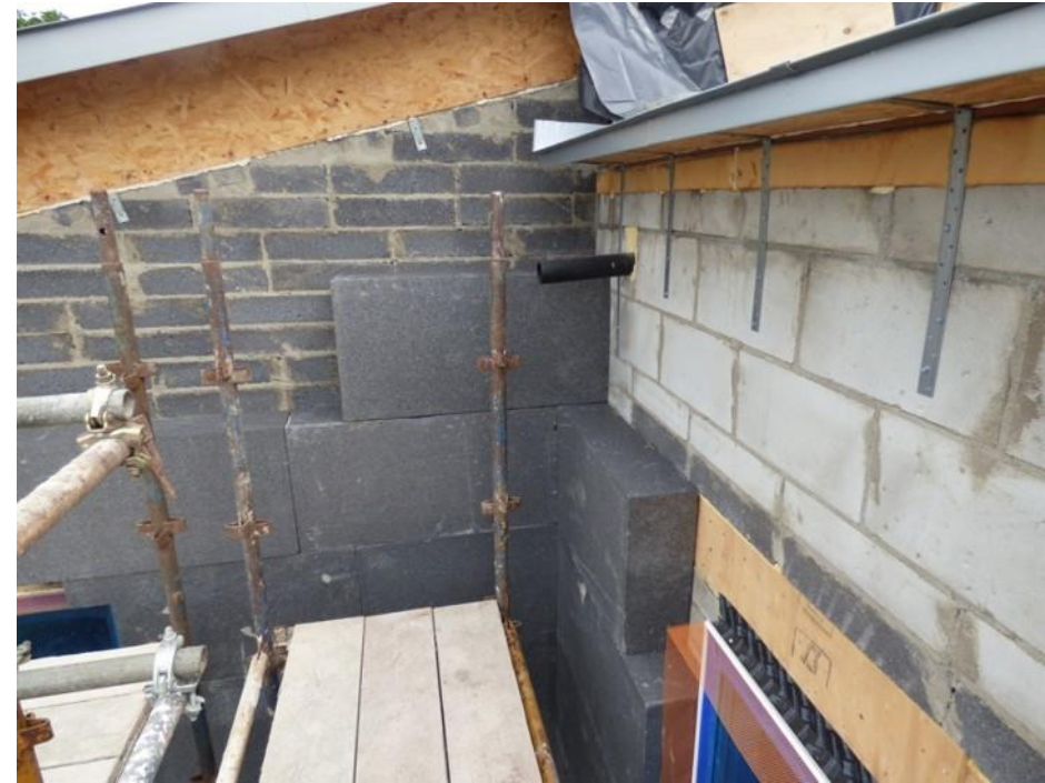
Tony's house walls with external insulation slabs.
